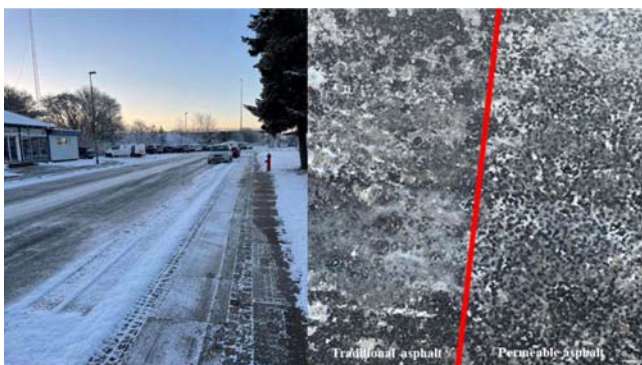
Fig. 7. Road 6 in December 2022, Where Ice Had Clogged the Pores (left) (The difference between a traditional pavement and a permeable pavement surface is shown on the right-hand picture. Photo was taken on 15.12.2022.)
