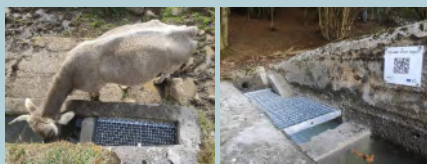
Compensatory measures: drinking trough repair (above) and cattle pens repair (below).
